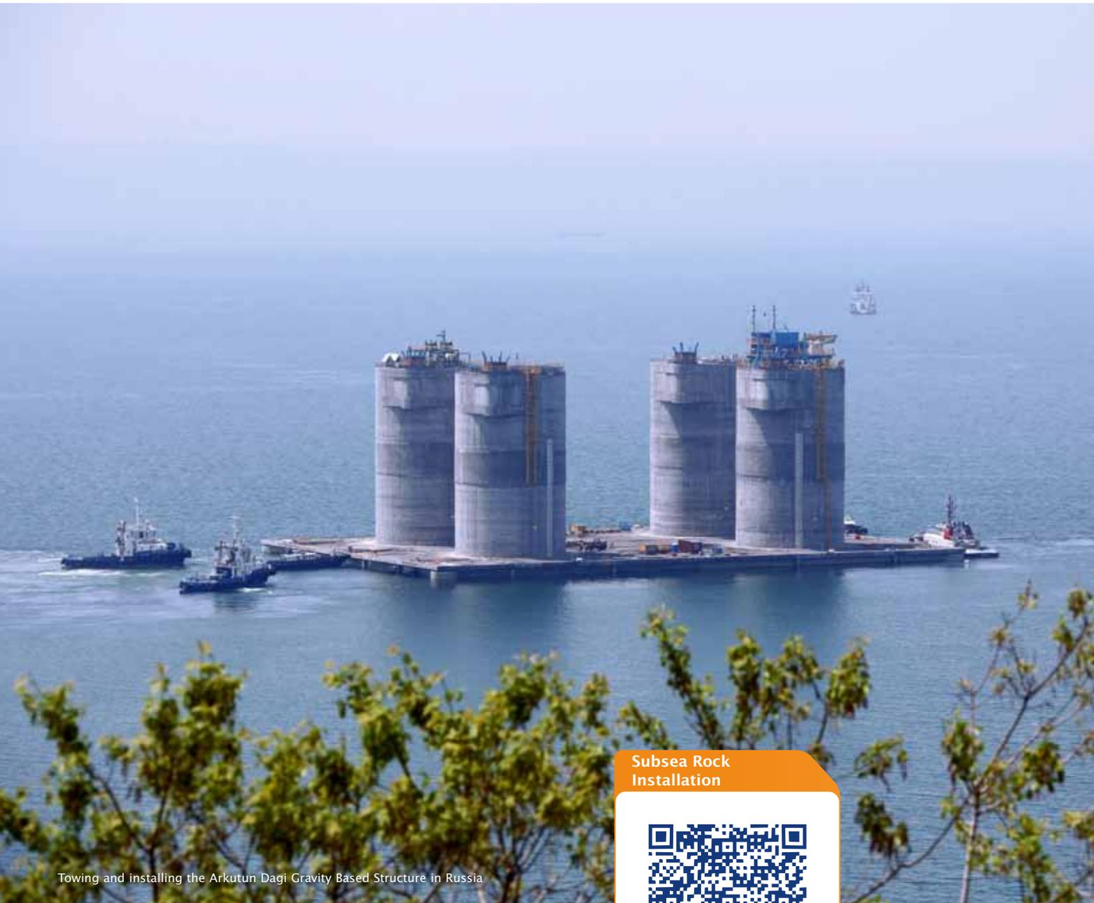
Towing and installing the Arkutun Dagi Gravity Based Structure in Russia
